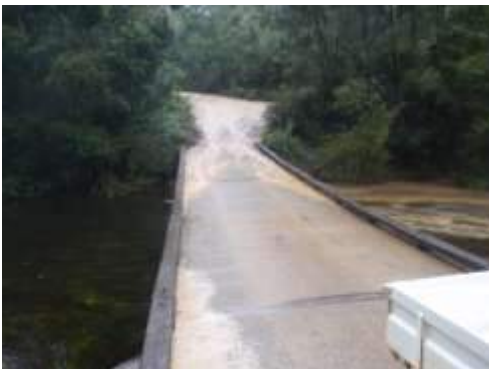
Sediment run-off into the Clyde River
