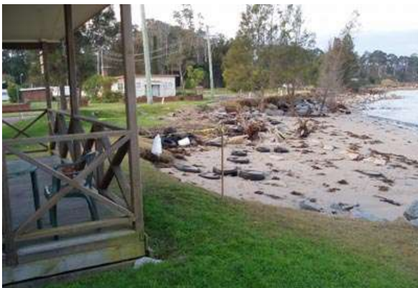
Erosion at Wharf Rd, Batemans Bay 2005
