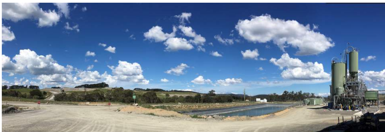
Figure 2. Panorama from processing plant area showing processing plant ponds of contaminated water in centre; mine access road and waste rock dump on skyline at left; the tailings dam wall behind the ponds.
