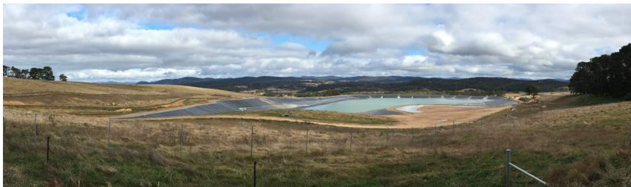
Figure 1. Tailings dam with tailings being discharged from a line of spigots on the far side on the inside of the dam wall; note narrow 'beaches' of exposed tailings; black material is the impervious liner; note bund (earth embankment) which diverts clean overland flow away from the dam; work is underway on the left hand side to raise the height of the containment.
