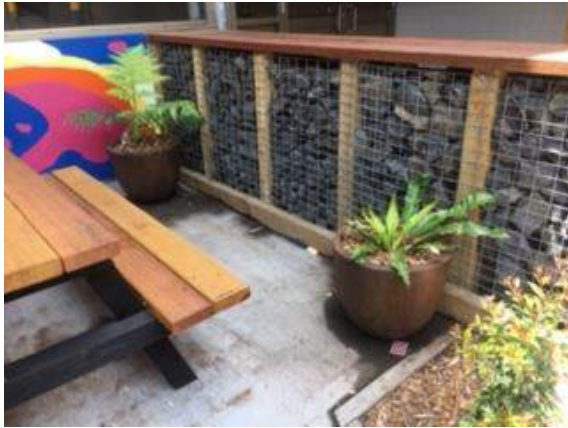
Above: Tree Fern and Birds Nest tubs established by SEC alongside picnic table and gabion wall constructed by Hands On Learning group.
